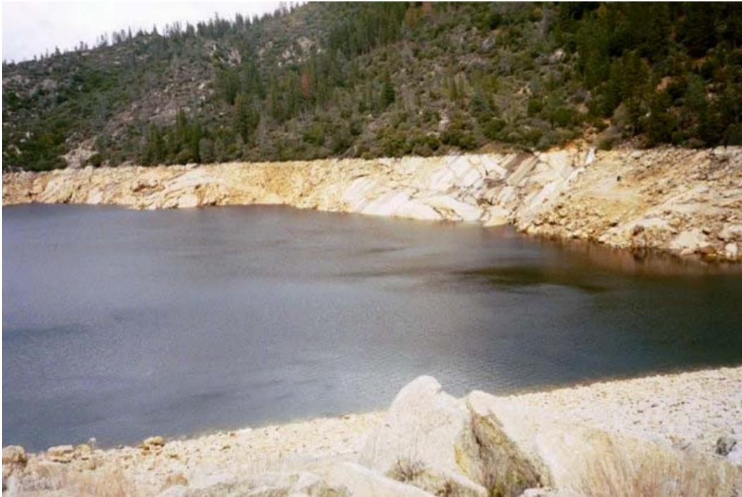
View of Mammoth Pool from Mammoth Pool Dam on April 14, 2003. This is an area of concern for debris build-up. No debris was detected.
