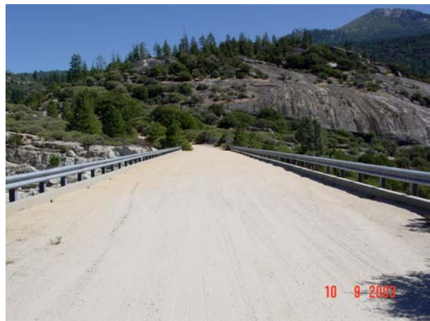
Sand placement on the dam to aid in deer crossing.
