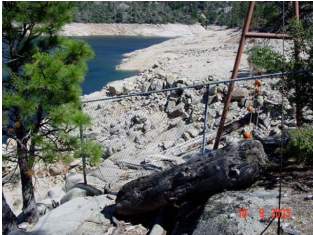
Fencing to spillway elevation along Mammoth Pool Reservoir and buoys across spillway.
