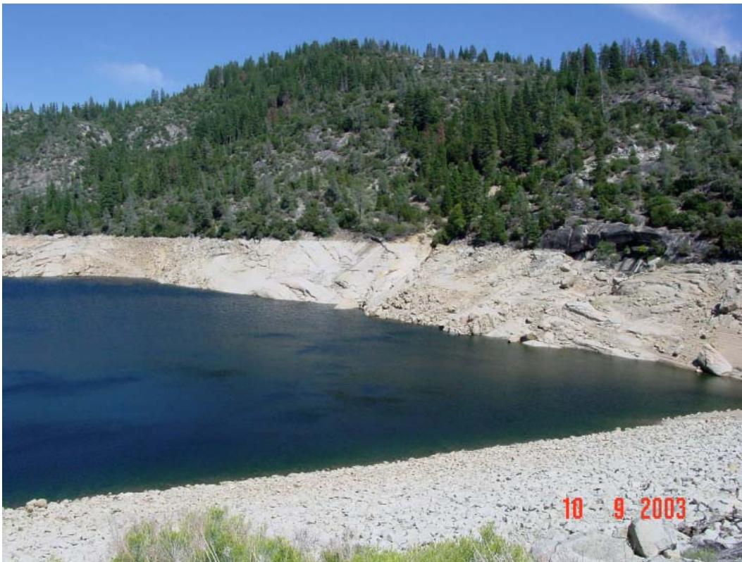
View of Mammoth Pool from Mammoth Pool Dam on September 10, 2003. This is an area of concern for debris build-up. No debris was detected.
