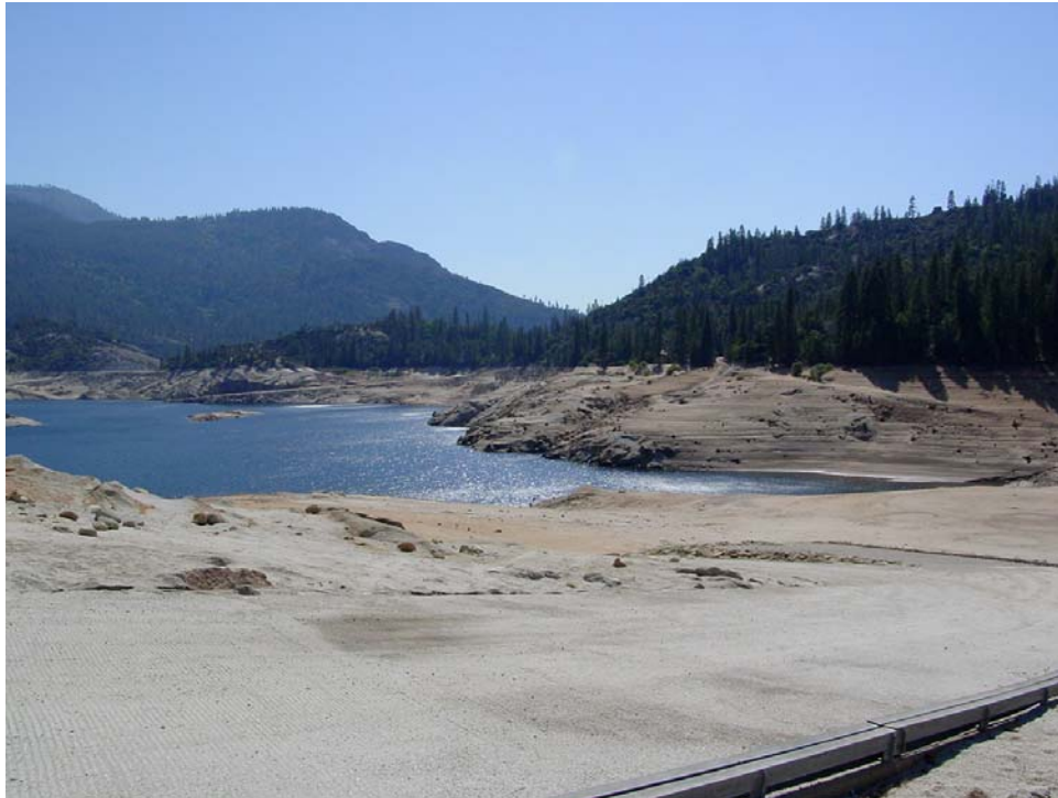
Mammoth Pool Reservoir Boat Ramp October 4, 2001, Reservoir 21% full
