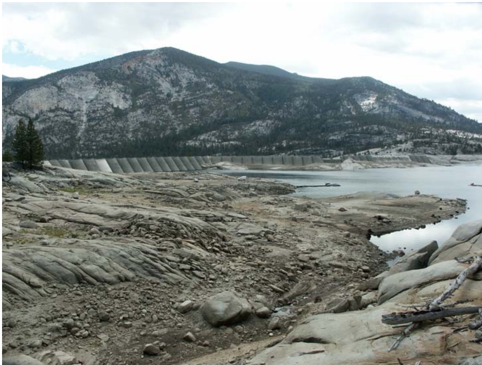
Florence Lake, looking at dam and Florence Lake Ferry Dock from work camp access road. September 4, 2002, Reservoir 31.1% full.
