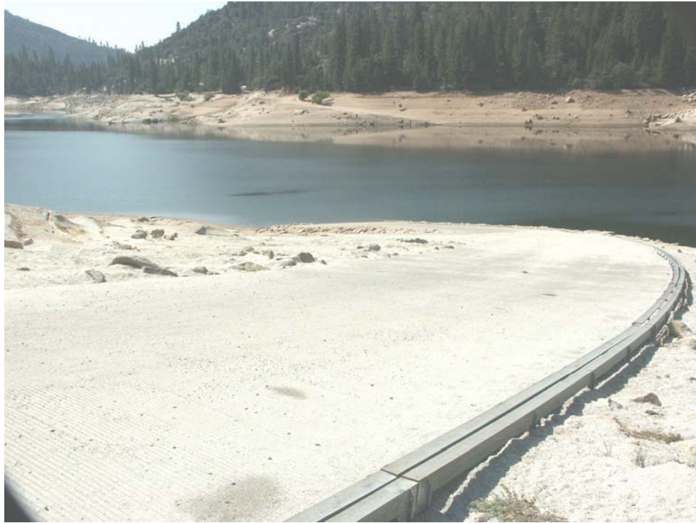
Mammoth Pool Reservoir Boat Ramp, looking S-SW August 29, 2002, Reservoir 54.7% full
