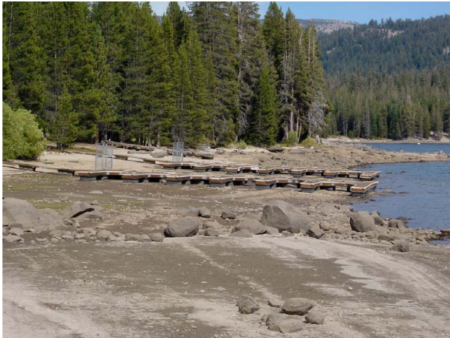
Huntington Lake Boat Ramp, looking south July 2, 2002 Reservoir 95% full
