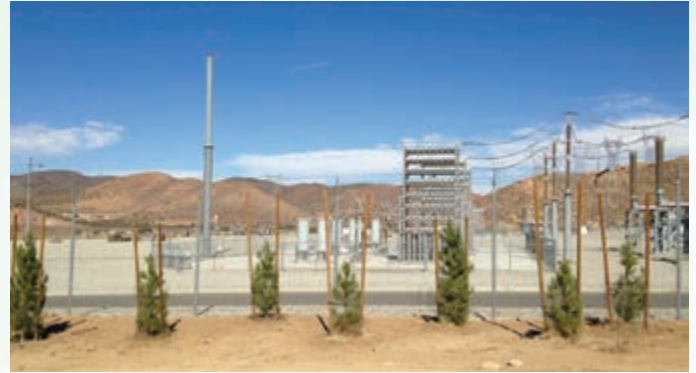
Earlier this year TRTP installed trees around the Vincent Substation.
