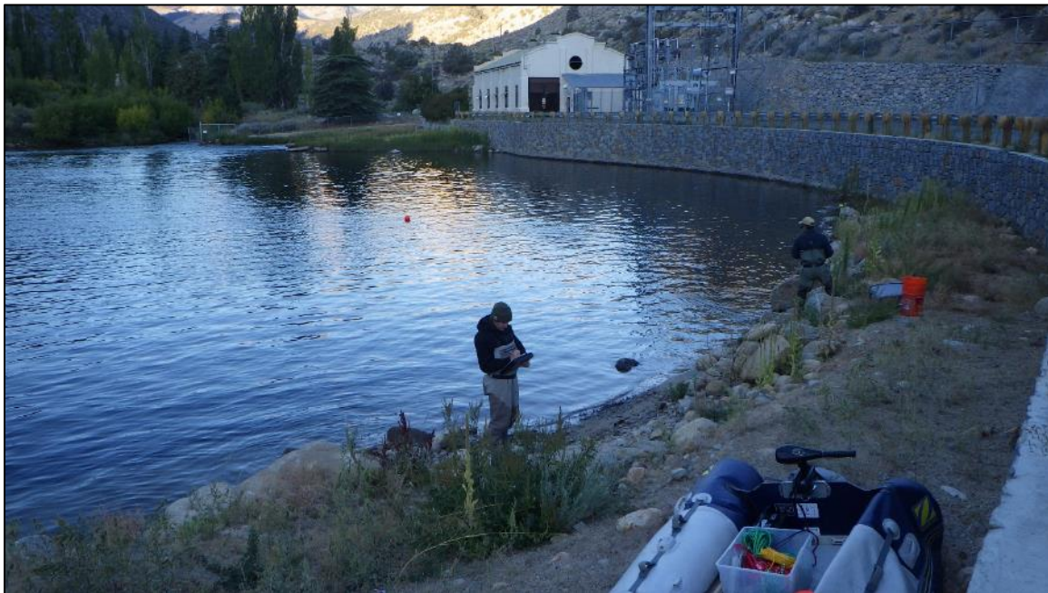
Figure A-37. Forebay 4 overview photo. September 24, 2019.
