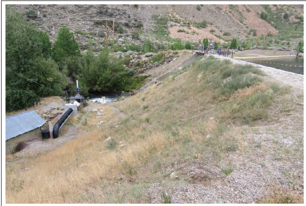
Photo 5: View of the dam and surrounding habitat at Intake No. 2.
