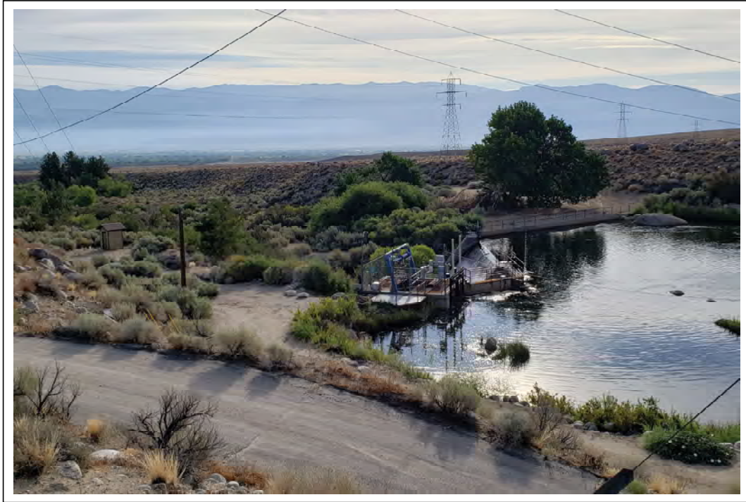
Photo 2: View of the dam and surrounding habitat at Powerhouse No. 5.
