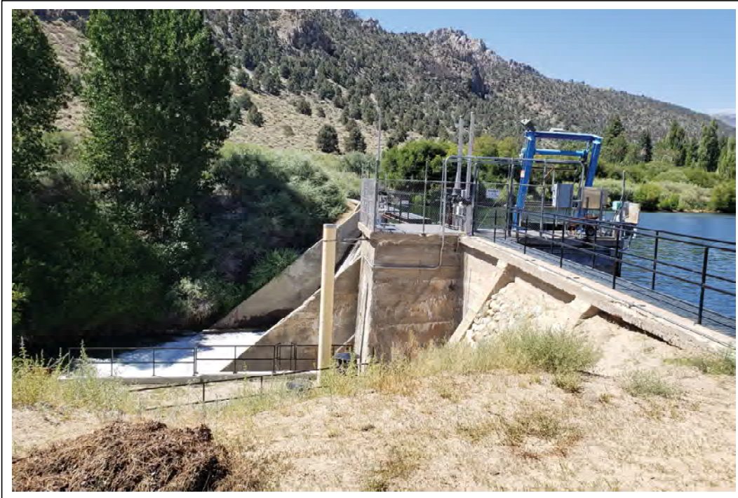
Photo 4: View of the dam and surrounding habitat at Powerhouse No. 3 and Intake No. 4.
