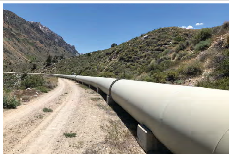
Photo 15: View of the flowline flowline road.
