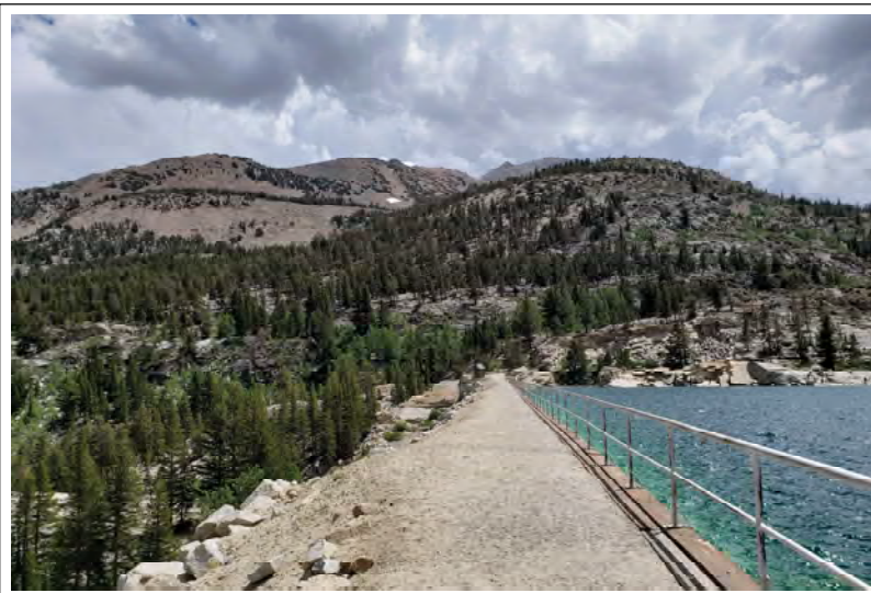
Photo 12: View of Hillside Dam and surrounding habitat at South Lake.
