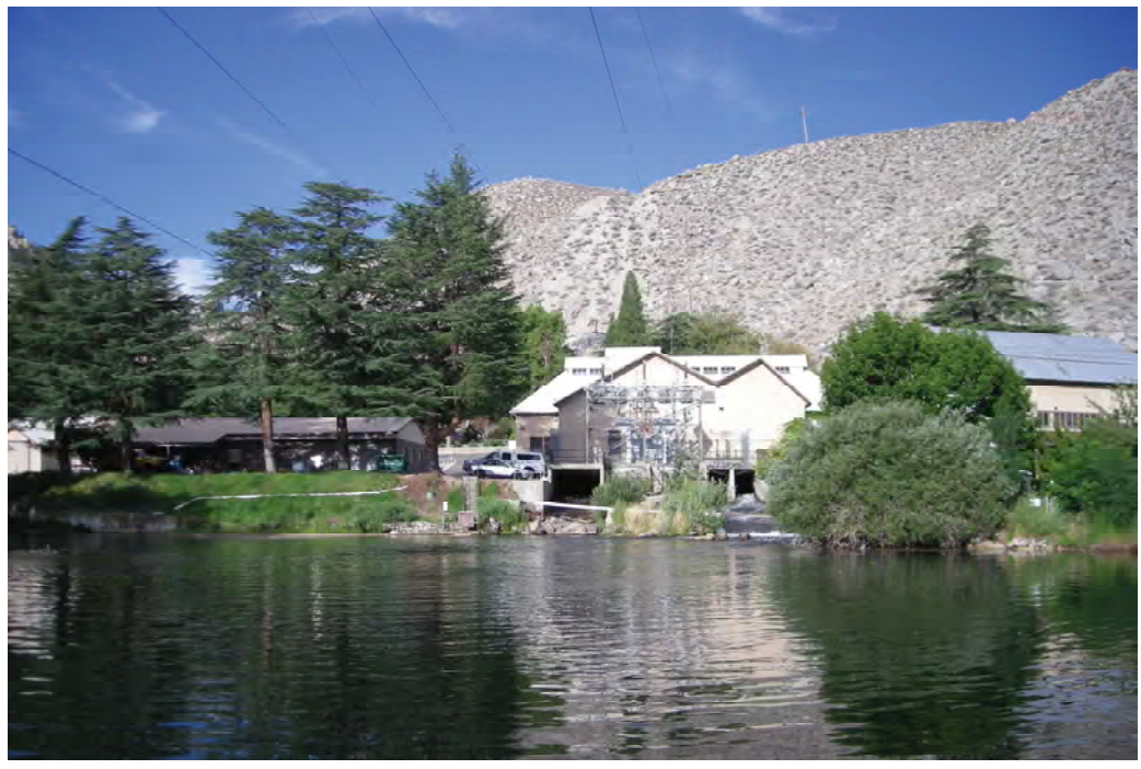
Photo 3: View of the dam and surrounding habitat at Powerhouse No. 4.
