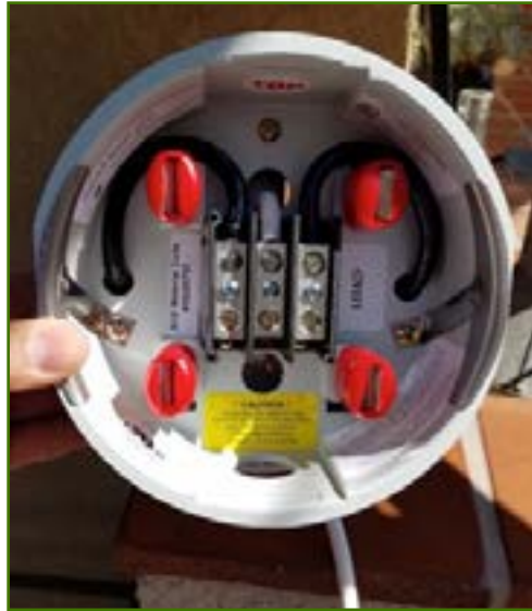
The internal Underside of the GMA
