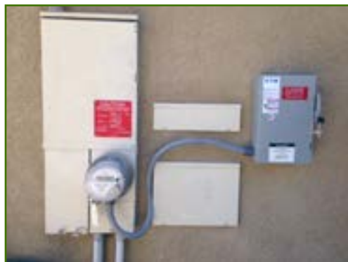
Securing a Flexible Conduit on the GMA Installation
