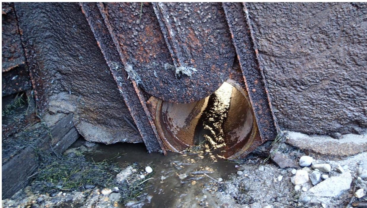
**Figure 4.1-1 Intake No. 5 Low-Level Outlet Slide Gate.**
