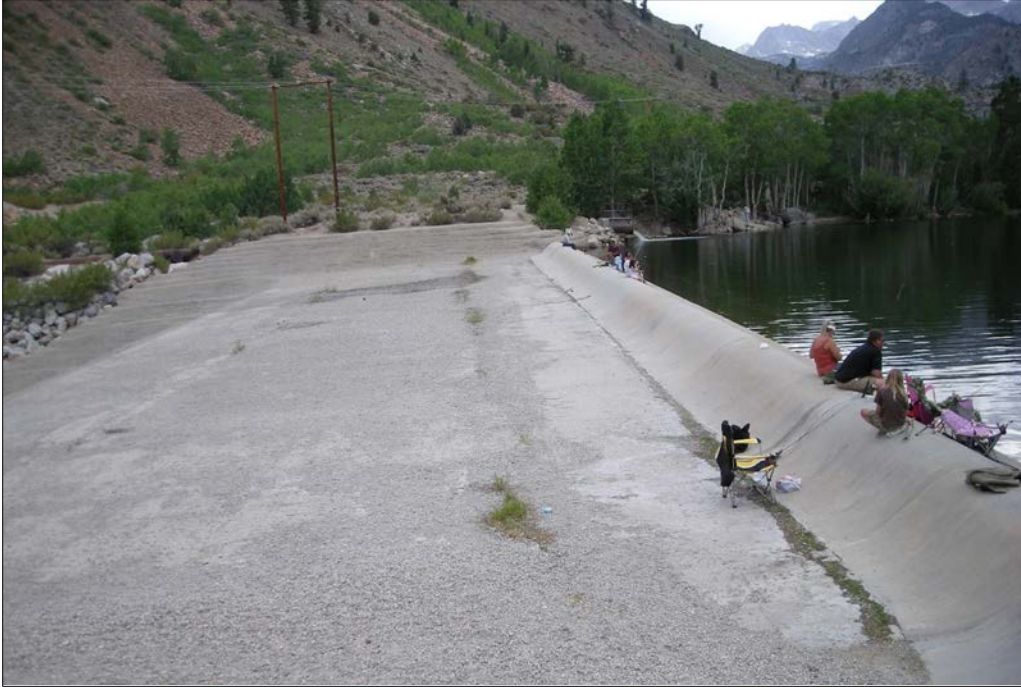
Photo 9.10-13. Intake No. 2 Dam and Spillway
