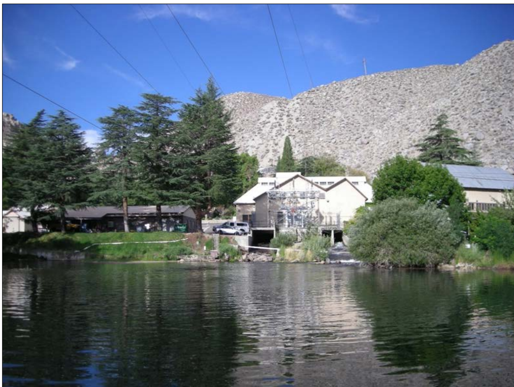
Photo 9.10-6. Plant No. 4/Intake No. 5
