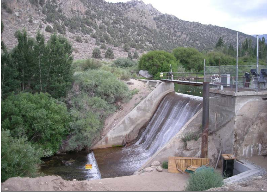
Photo 9.10-9. Plant No. 3 Spillway
