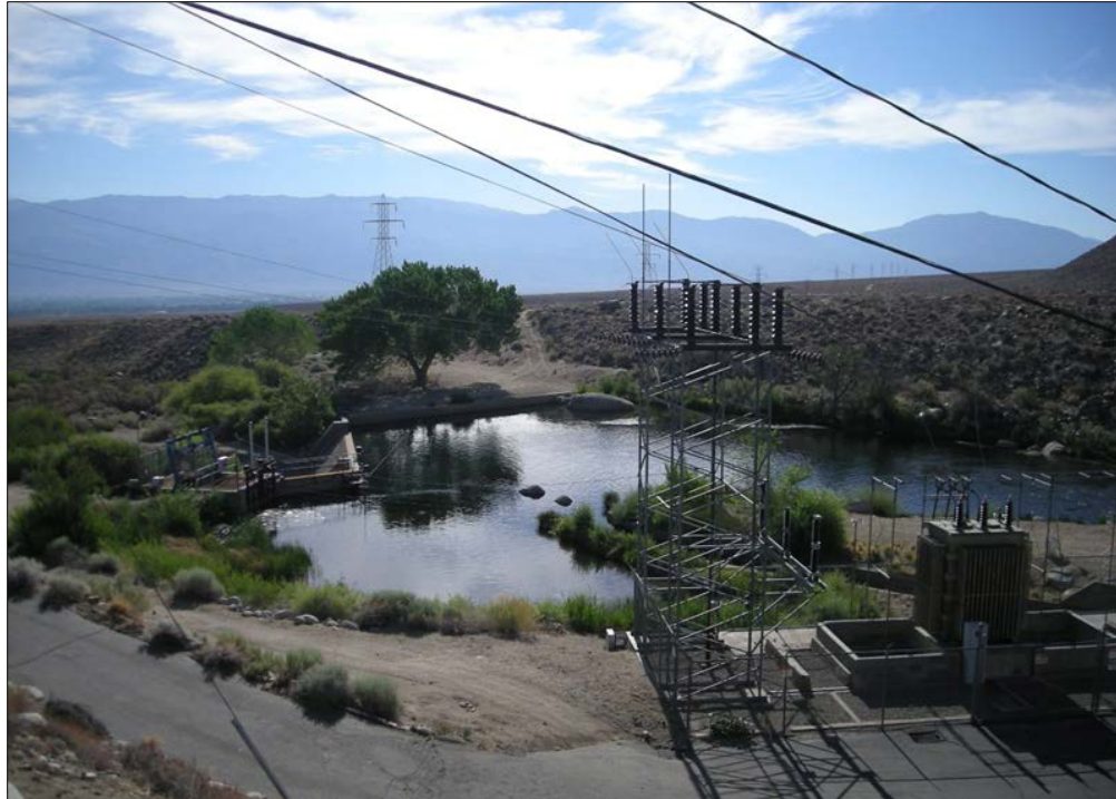
Photo 9.10-5. Plant No. 5 Facilities
