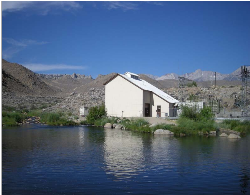
Photo 9.10-4. Plant No. 5/Intake No. 6
