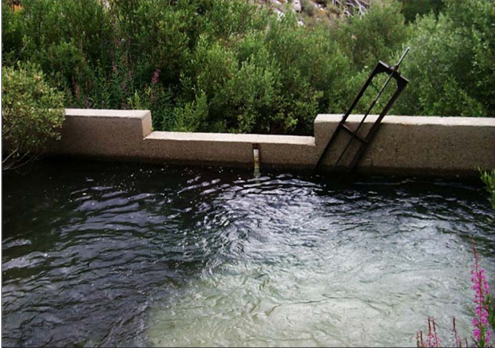
Photo 9.10-15. McGee Creek Diversion
