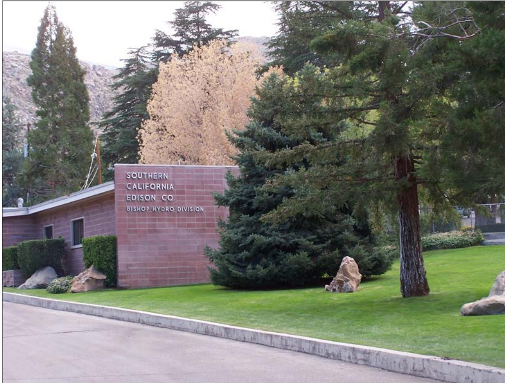
Photo 9.10-7. SCE Office at Plant No. 4
