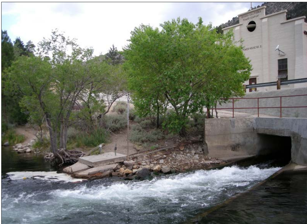
Photo 9.10-10. Plant No. 2 Facilities
