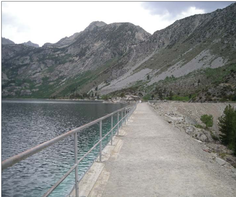
Photo 9.10-20. Lake Sabrina Dam
