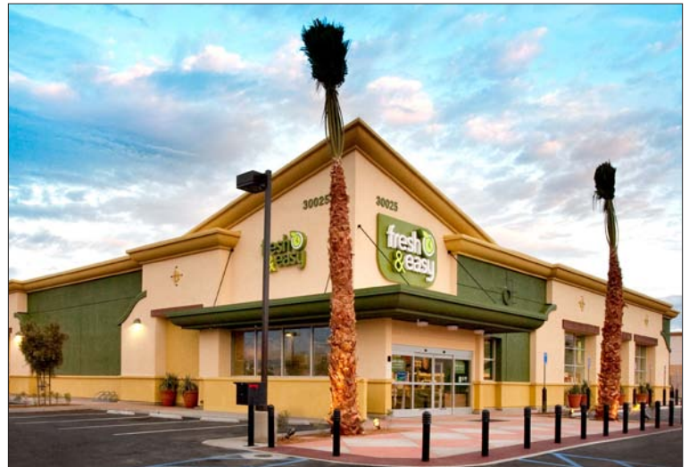
As part of an extensive commitment to energy management and sustainability, Fresh & Easy Neighborhood Markets work with SCE through the Savings By Design Program to receive design assistance and incentives for high-performance new building design and construction.
