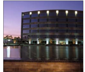
Eleven buildings at the Tri-City Corporate Centre in San Bernardino, including the Lakeside Tower (shown), can reduce load by 721 kilowatts during a demand response event under SCE's Auto Demand Response program.
