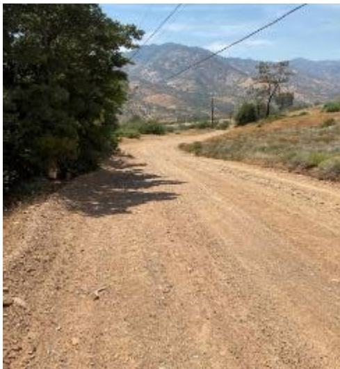
Left: Example of road in “Good Condition”
