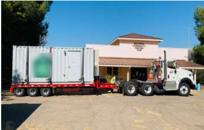
MBESS at community resource center
